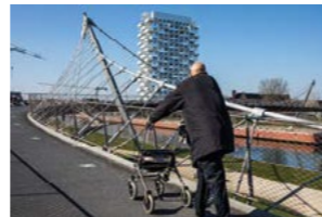
Collegebrug – Overleie, Kortrijk – Projectsubsidie 2012
