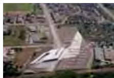
Parking & Terminus Hoenheim-Nord Zaha Hadid Architects 2001, Hoenheim
