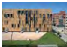
Carabanchel logements sociaux Foreign Office Architects (FOA) 2007, Madrid
